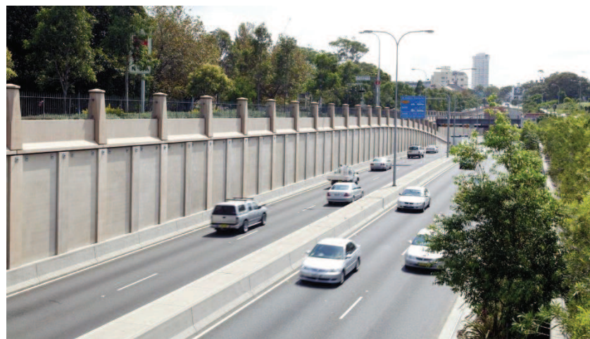
View of the four lane sunken Eastern Distributor with South Dowling Street operating up above
